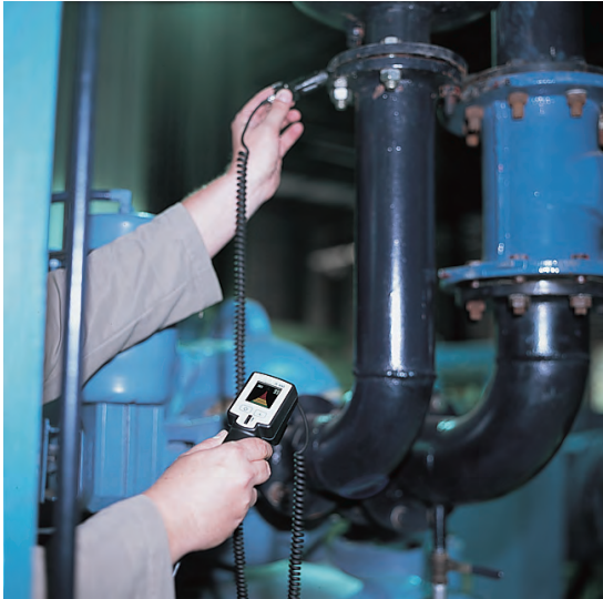
Leak detection with separated sensor
