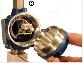
Unscrew the solenoid Housing threaded cap, By turning anti-clockwise
